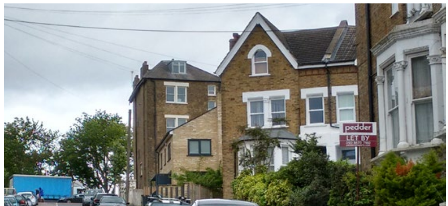
Front elevation of 1a Rockmount Road
