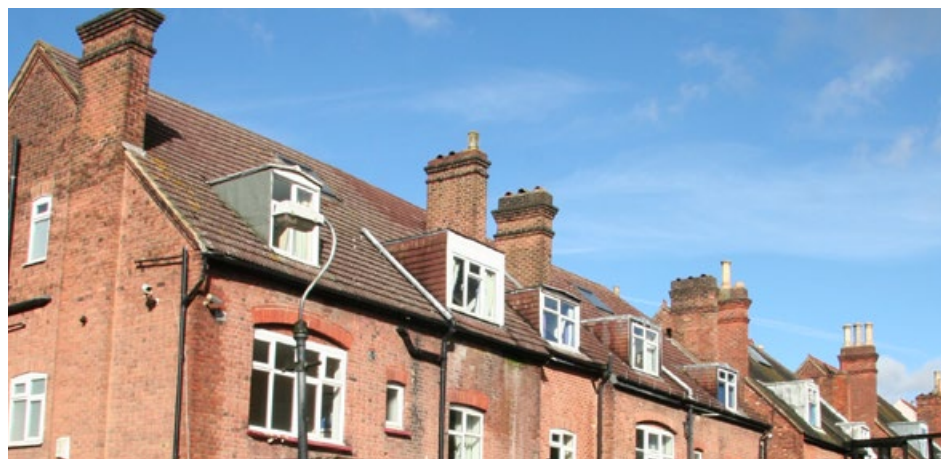
Addition of rear dormer windows breaking the rhythm of the original roof line
