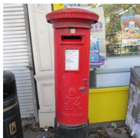
Historic letter box in need of maintenance
