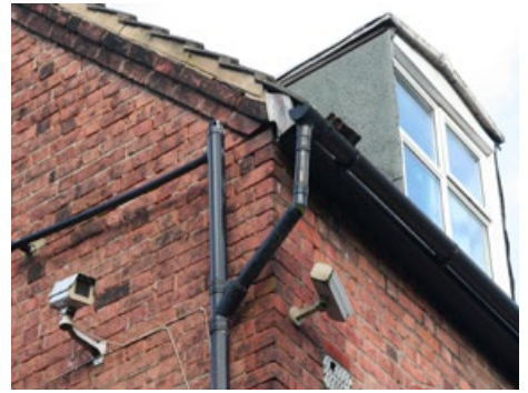
Poorly sited CCTV and unsympathetic dormer.
