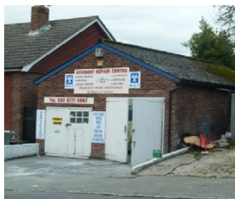
Accident Repair Centre
