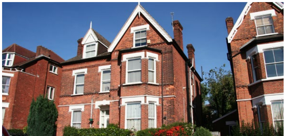
All traditional features are well maintained: Brickwork, timber sash windows, building plot, recessed porch, window lintels and timber barge boards
