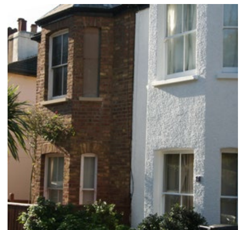
Original timber sash windows
