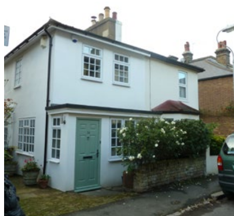
32-34 South Vale. Number 32 has an inappropriate front extension and uPVC windows
