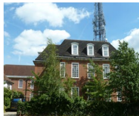
BT Telephone Exchange
