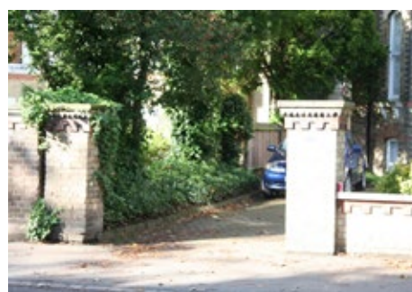
Typical street frontage opening between brick piers
