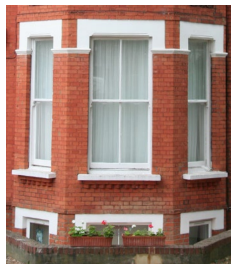
Original timber sash windows with lintel detailing above each window
