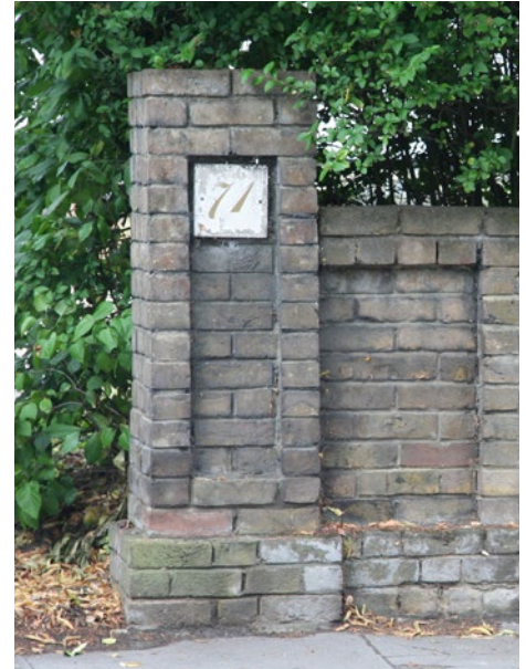
Example of brick wall boundary treatment
